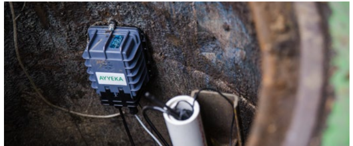
Installation of Wavelet Sewer Overflow Kit in San Francisco, CA.
