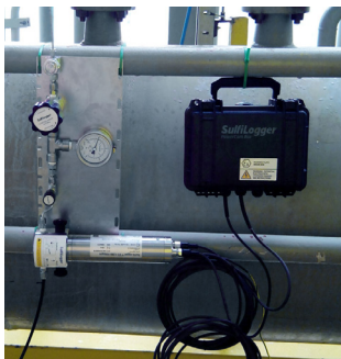
Flow cell (with flow & pressure control system)
